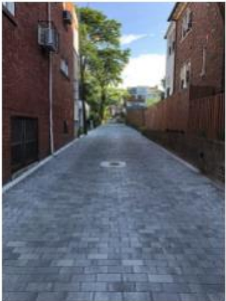
Parking lane permeable pavement
