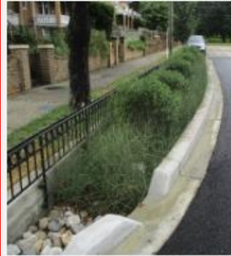
Curb extension bioretention
